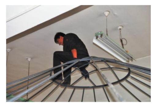
16) The crew using broomsticks help the **insulated top cover** move up the **rafters**. It will be a little heavy, it is insulated, and the larger the yurt, the heavier the cover. Be sure to have enough helpers on hand. >
