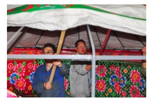
18) The hole in the **insulated top cover** needs to be centered over the outer ring of the **tono**. It isn't hard to do once it is on top of the **rafters**. >
