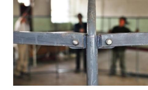
10) You can see here, a **rafter** slipped in the **wall support socket**. >
