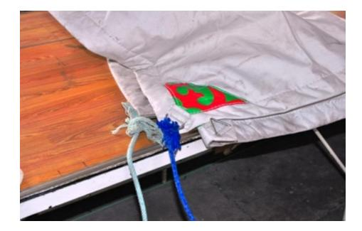
30) Some undone straps and buckles by the window. The outside window cover should roll up, with the material inward, toward the yurt so it will shed rather than collect water. The bug screen stays in place, but the inside plastic window can be zipped down. >
